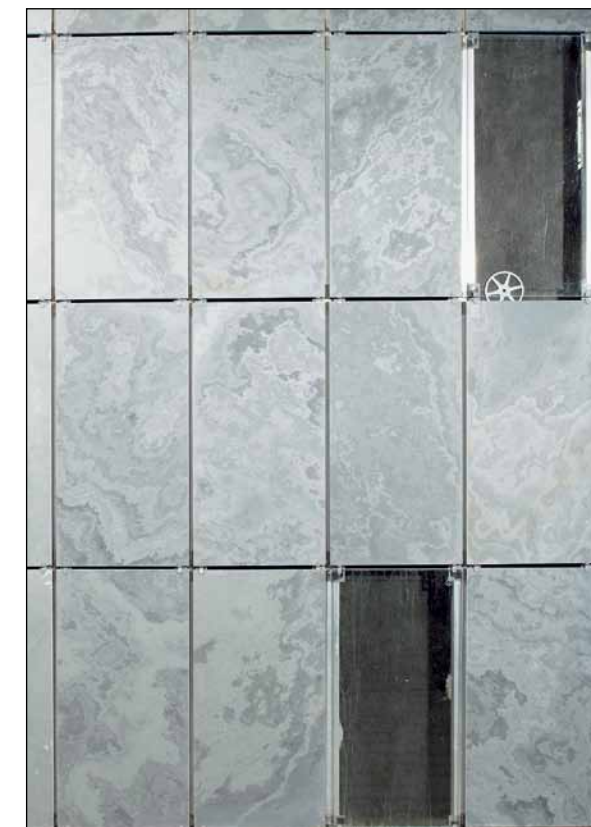
Symmetrical cladding 600 x 300 mm, laid vertically, fastened to the aluminium substructure with stainless steel mounting clips HE130
