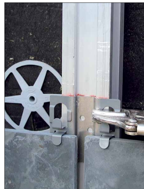
Symmetrical cladding 600 x 300 mm, laid vertically, fastened to the aluminium substructure with stainless steel mounting clips HE130
