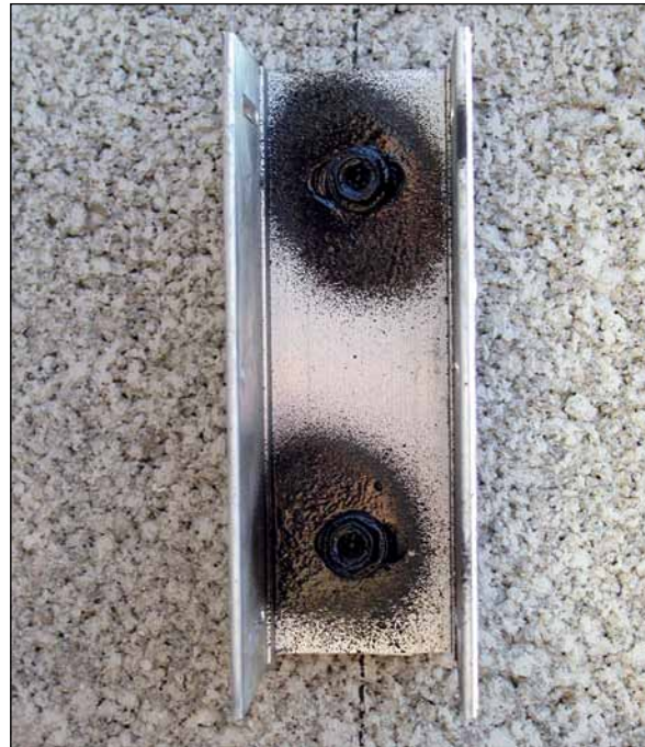
Teroson spray or similar (follow the specifications set by building inspectors)
