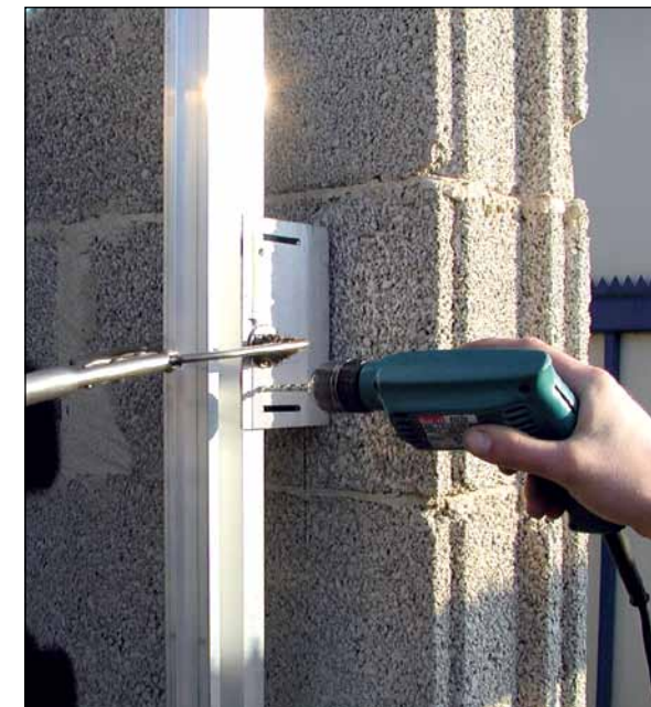
Hole diameter 5.2 mm
