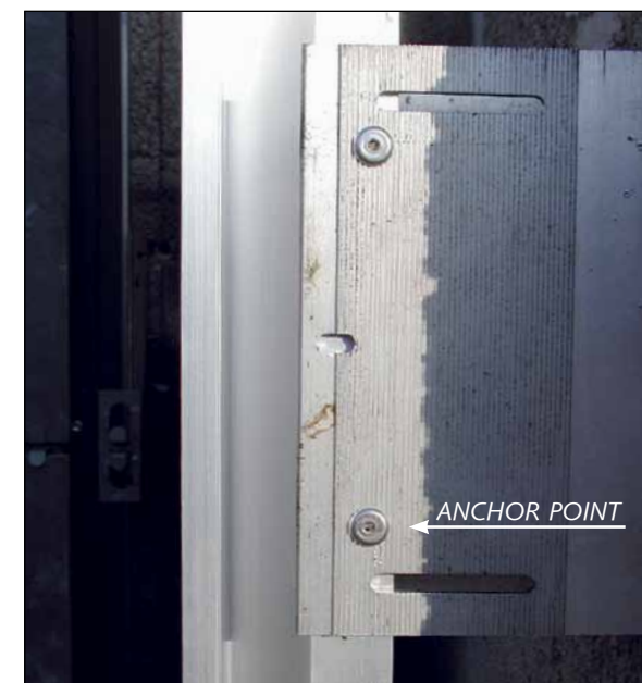
Hole diameter 5.2 mm
