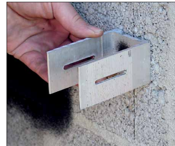
The slide point length is 50 mm. Also affix the slide point according to static specifications.
